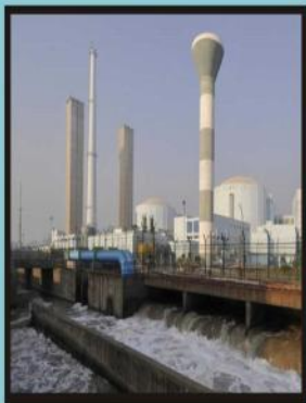
Tarapur Atomic Power Station
